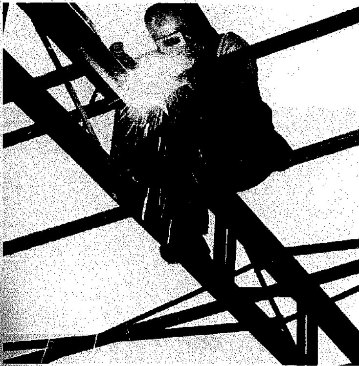
Much of the welding done in building construction is the shielded metal-arc process.
