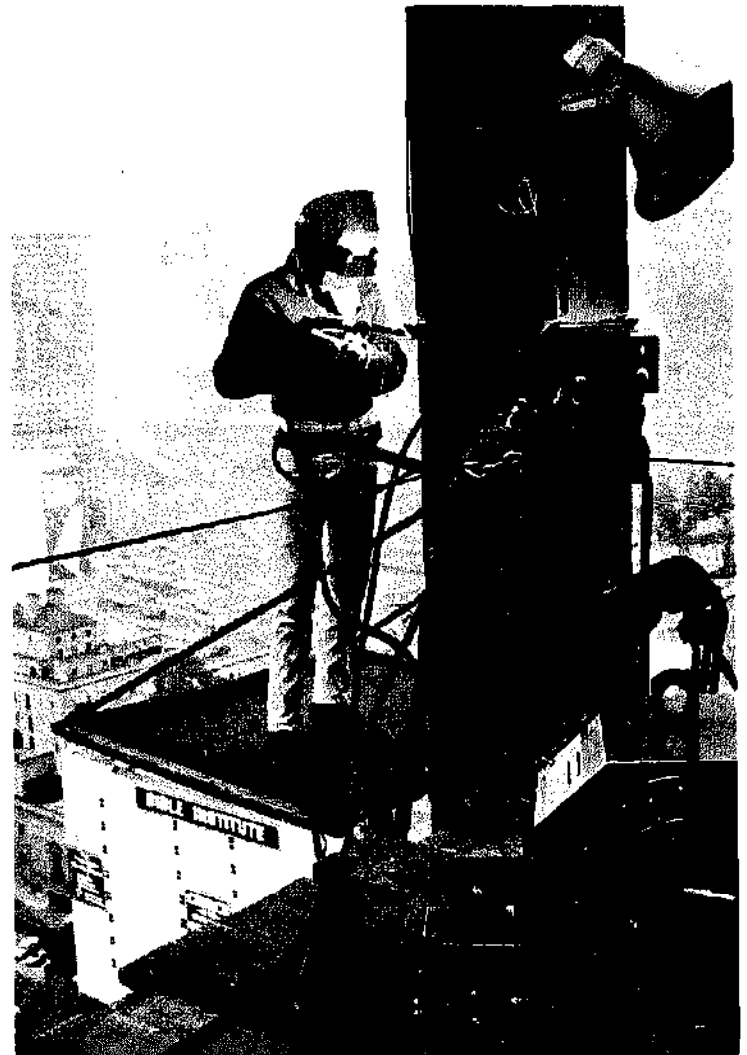
Fig. 1-14. Splicing a column during the erection of a building in Los Angeles, using the semiautomatic self-shielded, flux-cored arc-welding process.
