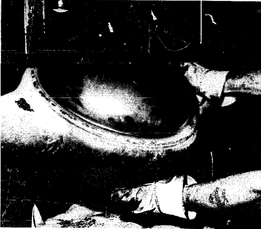
Visual inspection of this self-shielded flux-cored electrode automatic weld indicates good quality.
