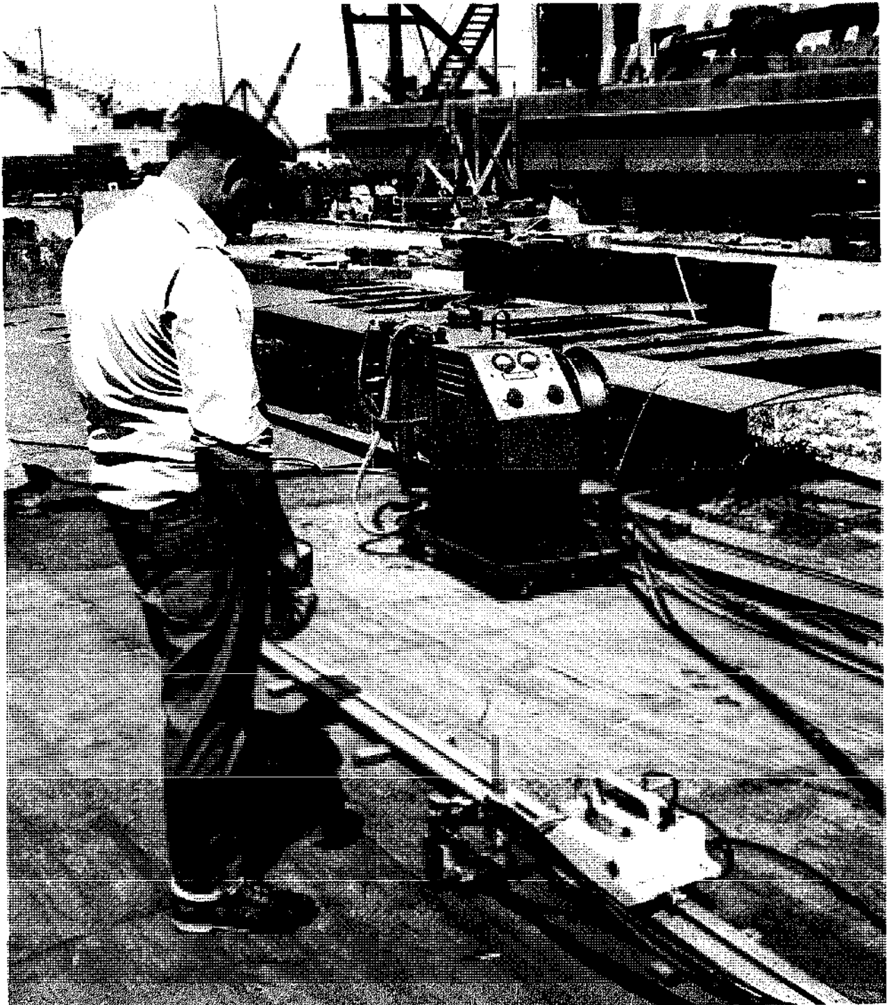
Splicing deck plate with mechanized submerged arc welding. Mechanized welding is an aid to minimize distortion.
