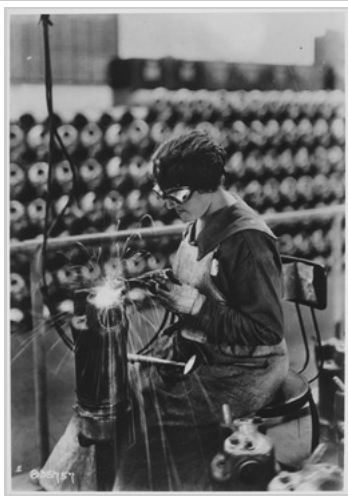
Acetylene welding on cylinder water jacket, 1918
