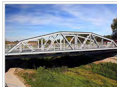
Bridge of Maurzyce
