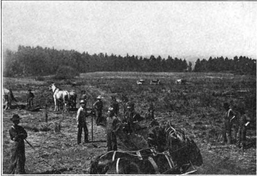
FIG. 103. — Mosquito control work on a large scale. Permanent corrective work, — draining a large pond in the background. Salt marsh work in California.
