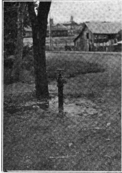
FIG. 97. — The leaking faucet with the resulting pool of water is often a constant menace in the entire absence of other mosquito-breeding sources.
