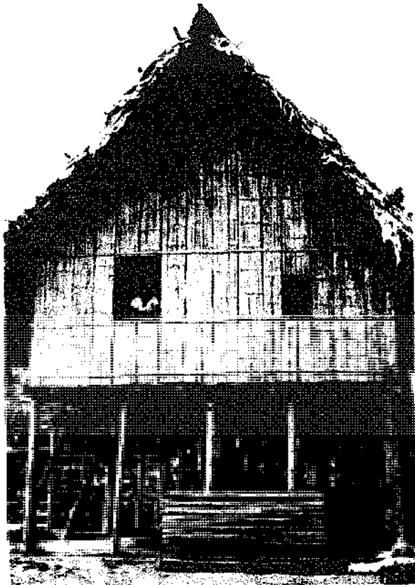
FIGURE 1--From supporting posts to rafters and sheathing, this cottage in the Ecuadoran lowlands is made entirely of native bamboo, Guadua angustifolia . The posts may serve for five years; the siding may remain in serviceable condition for decades.
