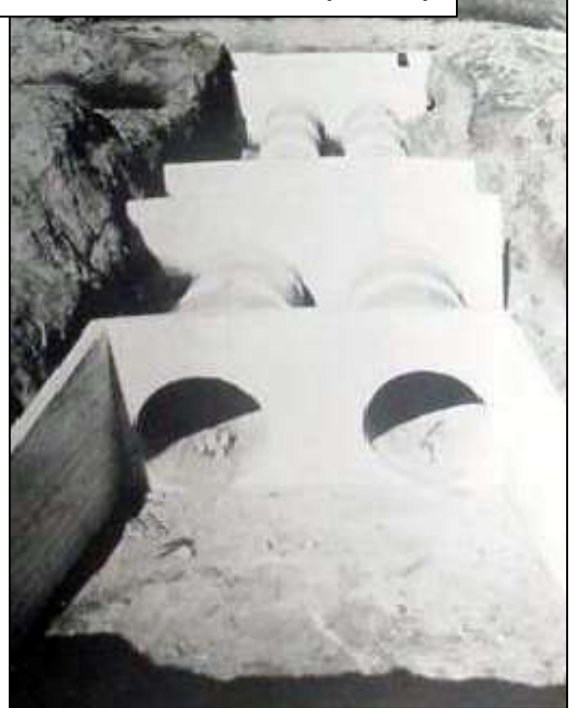
Culvert with collars (USBR)
