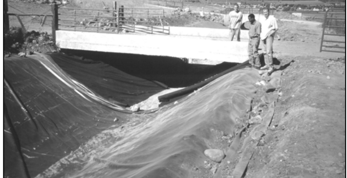
Installing plastic canal lining (courtesy R.W. Hill)
