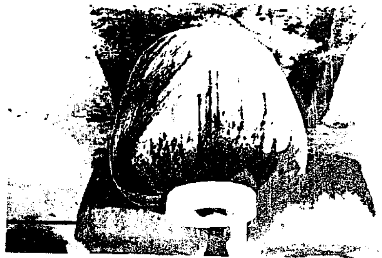
2.7 Place a circular ring on the top of the sack to make a mold for the opening of the jar. This can be made of wood or precast mortar.
