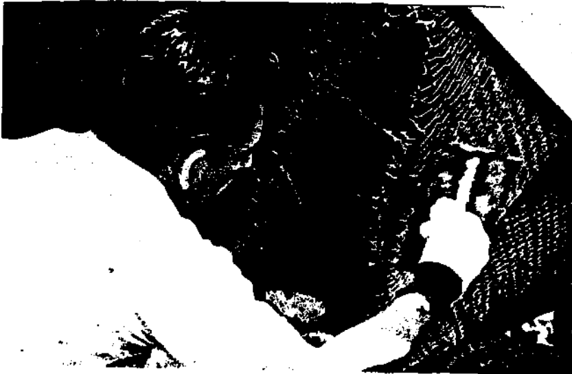
FIGURE 10 ... or trowel. The mortar is dry enough to remain in place when applied; a formwork is not needed. (Noel D. Vietmeyer, National Academy of Sciences)
