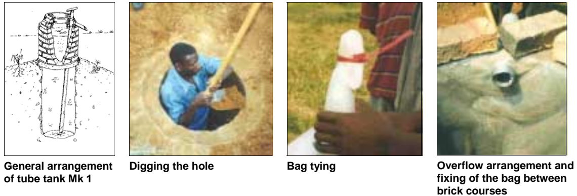
Figure 2.3: Original tube tank design. (all pictures from (Rees & Whitehead, 2000))
