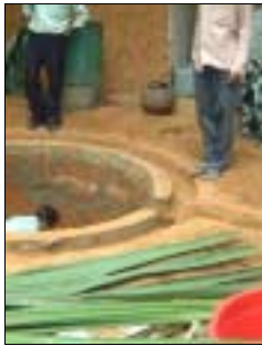
Ring beam with trench
