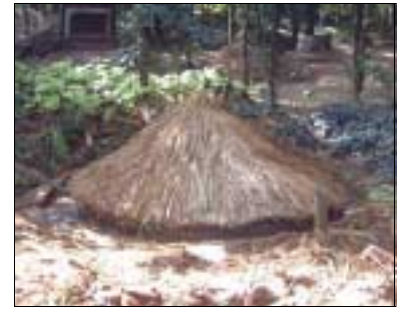
Finished tank with cover in place
