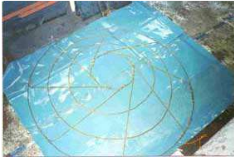
Figure 7. The frame with hoops in place.
