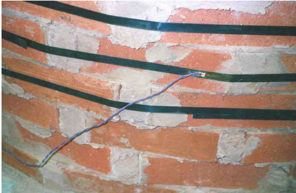
Figure 7 – Showing strain gauge fitted to the steel strap
