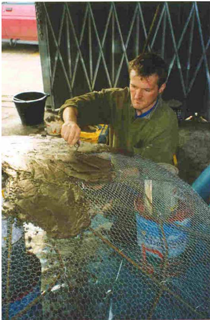
Figure 12. Applying render to the chicken mesh.
