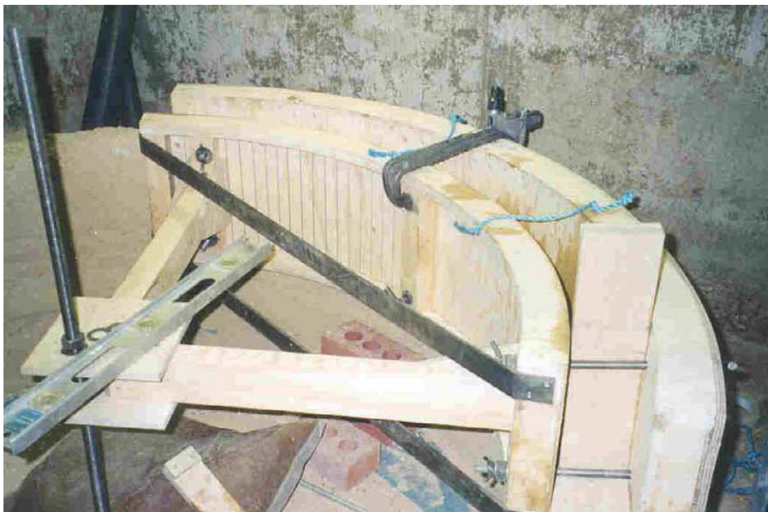
Figure 7 – Revised shuttering arrangement shown during construction of the experimental tank
