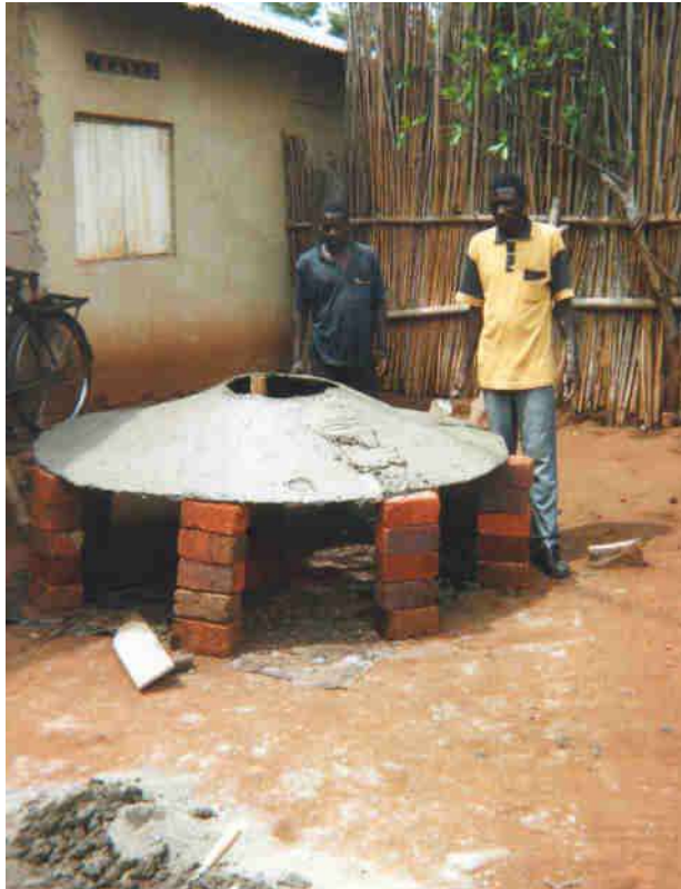
Figure 2 – A thin shell ferrocement cover near completion and ready for fitting to a PBG tank
