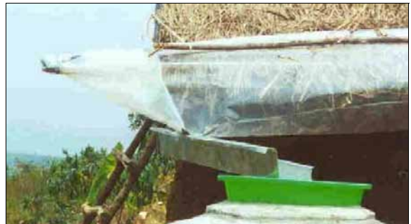
Figure 8.1: Plastic sheet guttering
