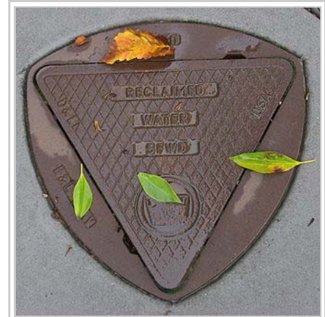
Cover for reclaimed water valve, San Francisco Water District
