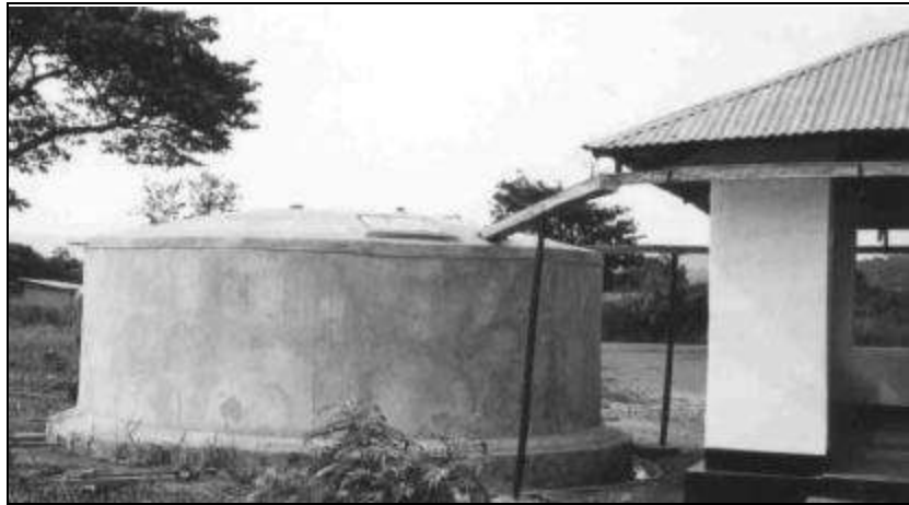
Fig. 1.2 A 46m^3 community ferrocement storage tank in Uganda
