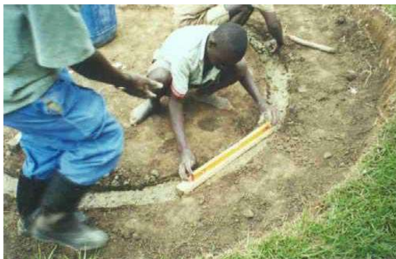
Figure 3 - Casting the ring beam
