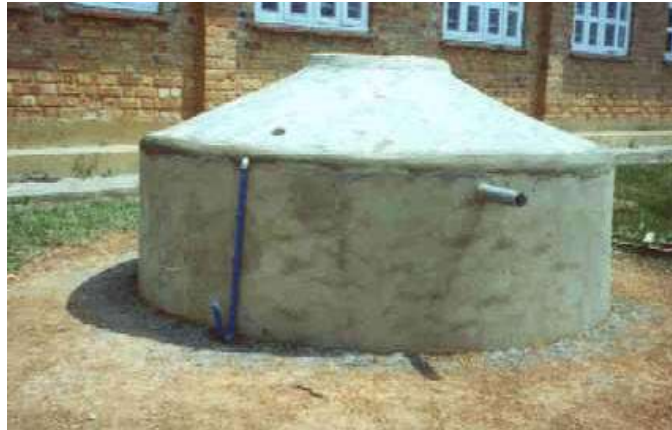
Figure 13 - The tank with cover in place
