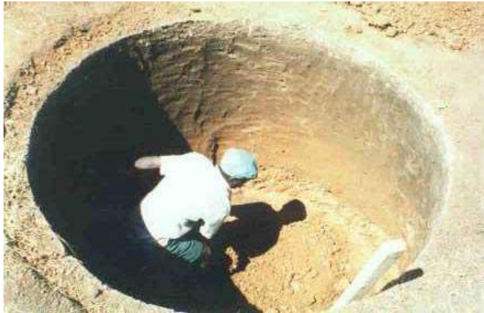
Figure 5 – Excavation of the tank
