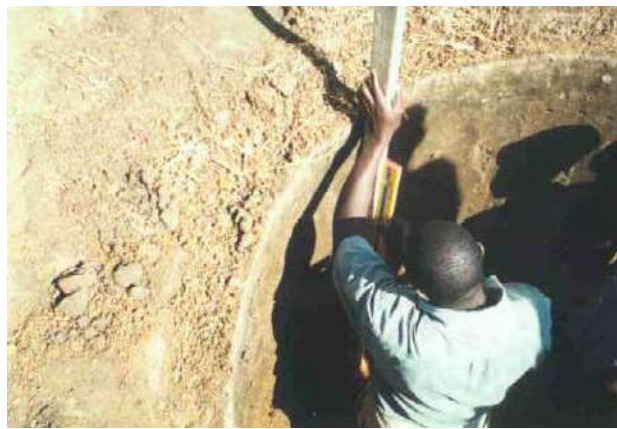
Figure 6 - Plumbing the walls to keep them vertical
