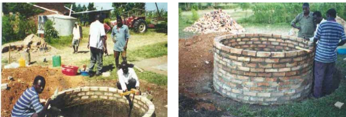
Figure 10 - showing the construction of the parapet wall
