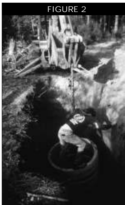
A shallow well may be dug with a backhoe.
