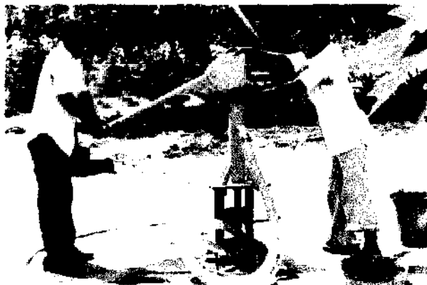
Fig. 182. For the disinfection of a well the pumped water is recirculated into the well.
