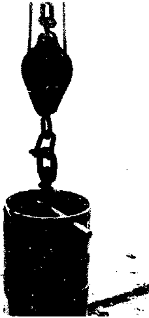
Fig. 168. The casing hanging from the hook. Note that for this heavy job both pulley wheels of the upper block are used (compare with Figure 159).
