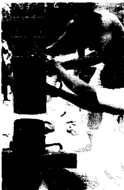
Fig. 69. A casing section ready to be screwed onto the previous one.
