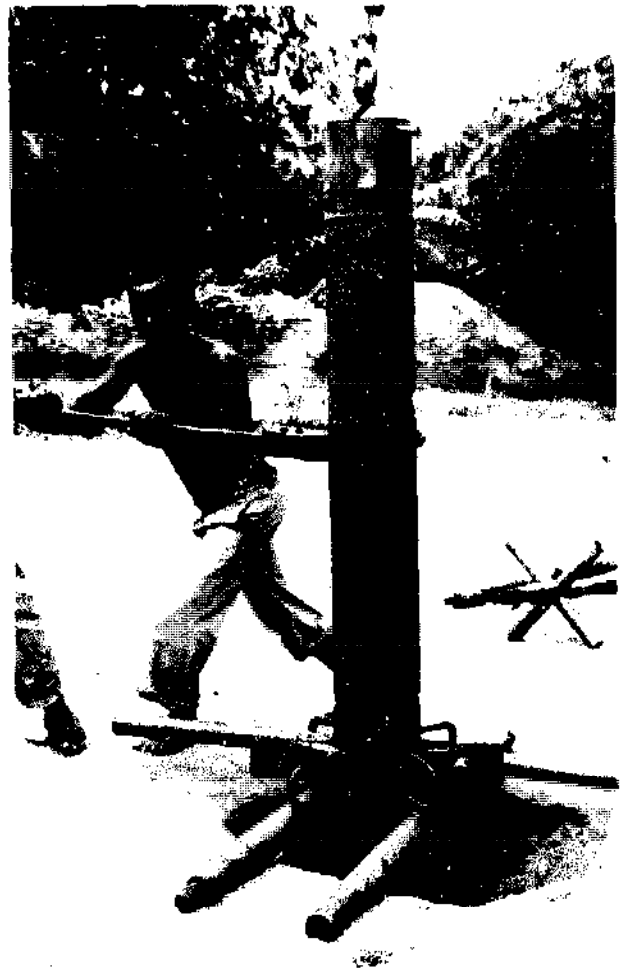
Fig. 89. Casing sections are unscrewed by means of a chain spanner.
