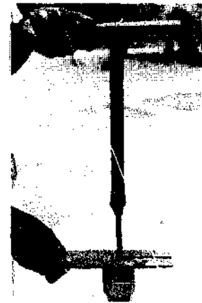
Fig. 128. Pumprod puller and catcher.
