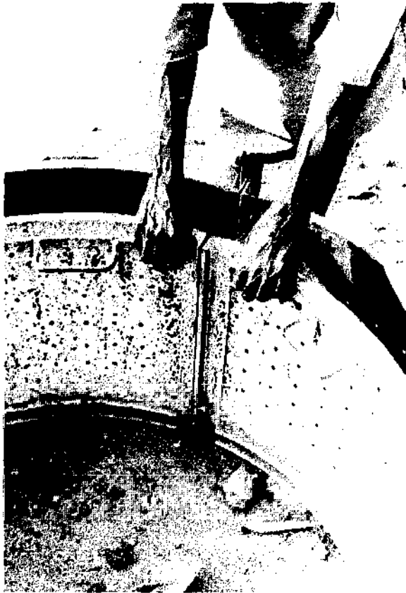
Photo 22 Caisson ring mould 0.5 metre deep -- a) Interior sections. -- Upper Volta.
