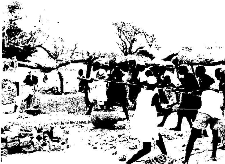
Photo 35 Lowering man down the well. The improvised headframe is made from local timber. – Upper Volta.
