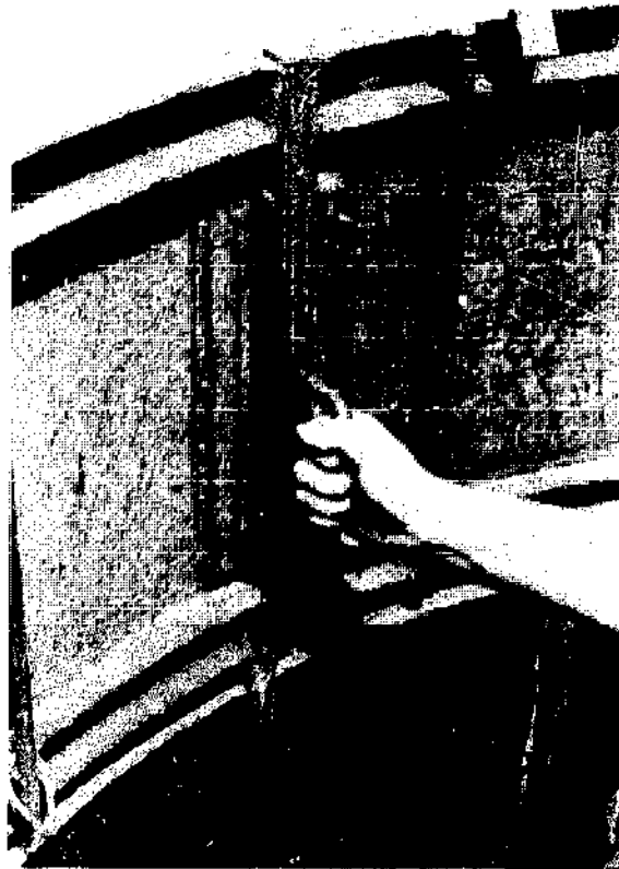
Photo 13 d) Shutter wedge, these are unbolted and pulled out to release shutters from well.
