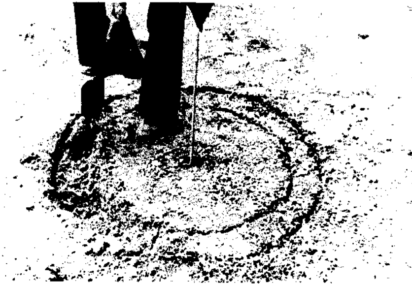
Photo 60 Making the Cutting Ring Without a Mould — a) Mark out ring on ground and dig roughly to size.
