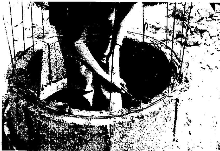
Photo 72 f) On every course of blocks a horizontal re-rod is tied, laid on a bed of mortar and the next row of blocks laid.
