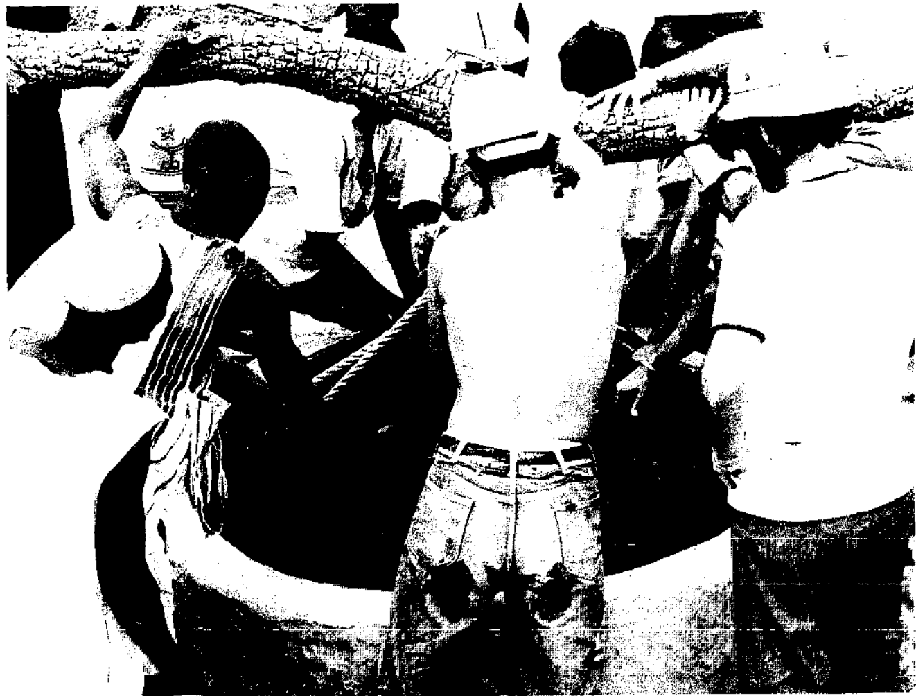
Photo 54 f) Lower assembled sections into well. – Upper Volta.
