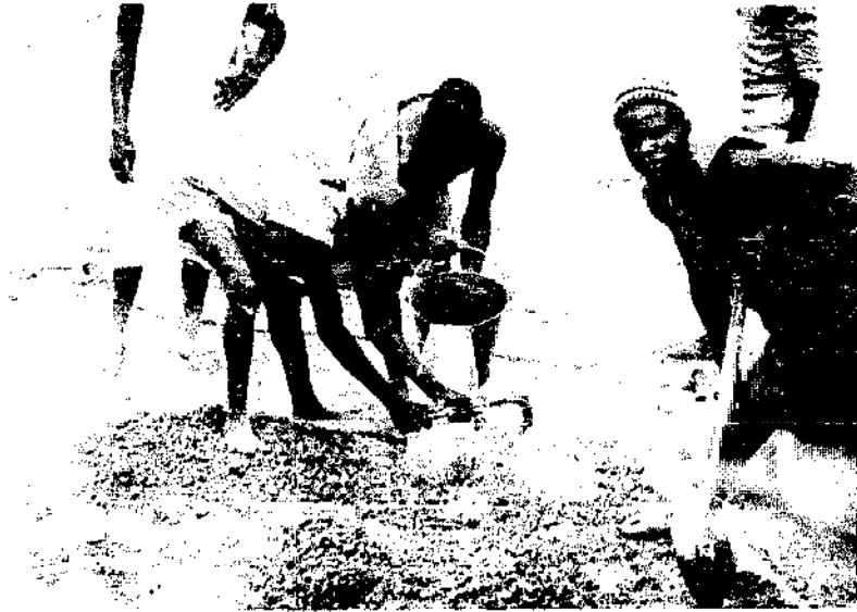
Photo 14 Mixing the Concrete by Hand on the Mixing Tray – Low walls prevent accidental loss of cement slurry. In the photograph a hoe is being used; square shovels make the work easier. – Upper Volta.
