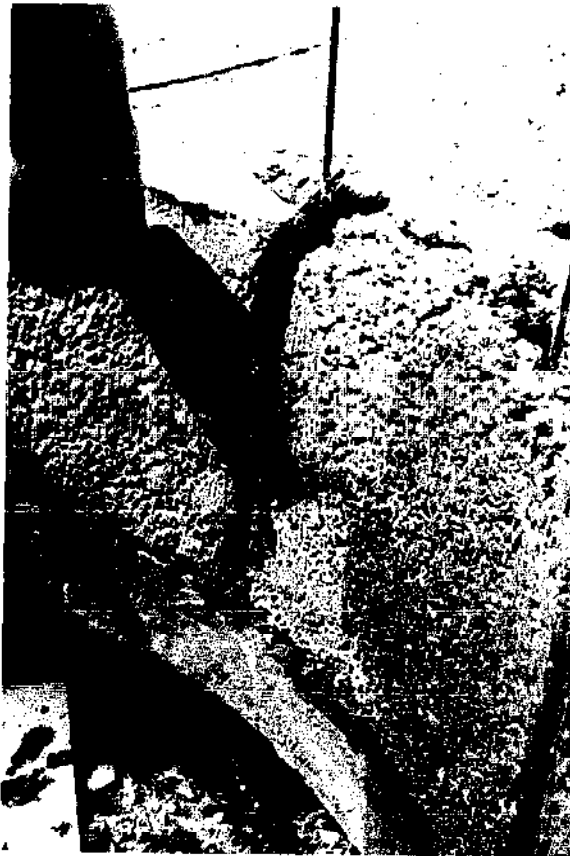
Photo 71 Using Porous Concrete Blocks for Caisson Sinking – e) Trowel mortar into gaps between blocks and fill cut-outs around re-rod with mortar.
