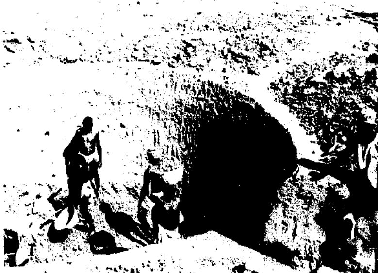
Photo 4 d) Excavating 10 metre diameter well and removing spoil up a ramp cut into the side of the well. Well excavated into slow flowing aquifer. — India.
