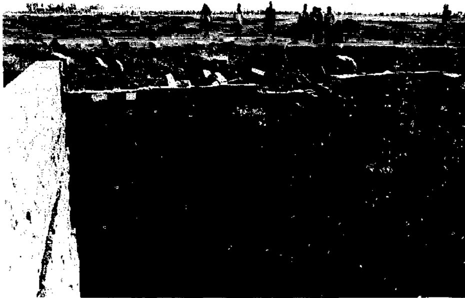
Photo 2 Large Oversize Hand Dug Wells b) Masonry lined, 15 metre square well, with steps for access. — India
