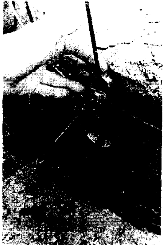
Photo 65 f) Fill mould with concrete and tamp to consolidate and remove air bubbles. (left)
