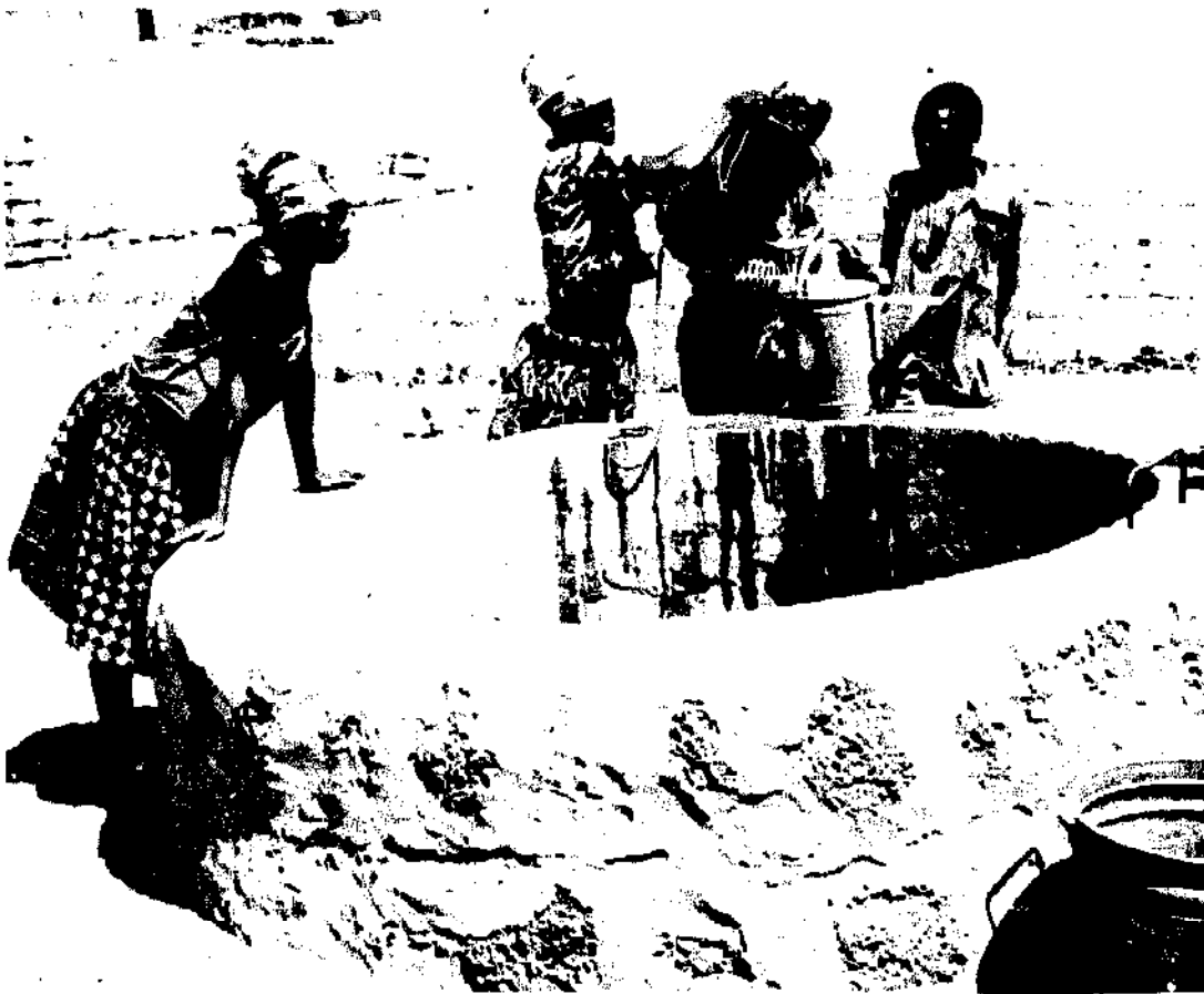
Photo 45 Masonry Lined Well – Upper Volta.
