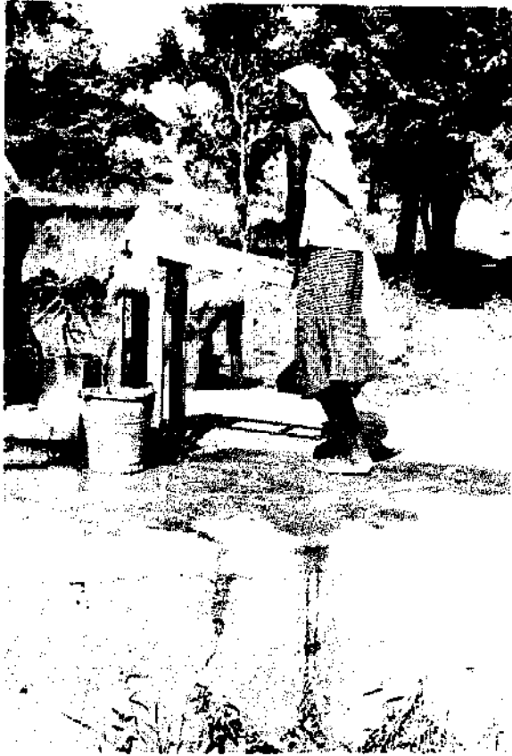
Photo 87 Improved Water Well Pumps — a) 'Abi' type pump made overstrength to withstand constant use. This pump is expensive but is an improvement on the standard commercial types. — Senegal.
