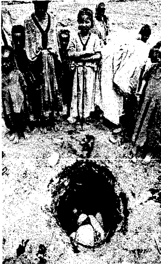
Photo 8 Wellhead Contamination – c) Hand dug well used for water supply. The mouth is lined with loose stone blocks but polluted surface water and rubbish can enter the well. – Upper Volta
