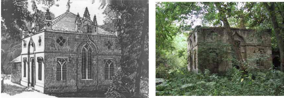
Fig. 24 Howsham Mill c.1945 (32) Fig. 25 Howsham Mill before renovation (32)
