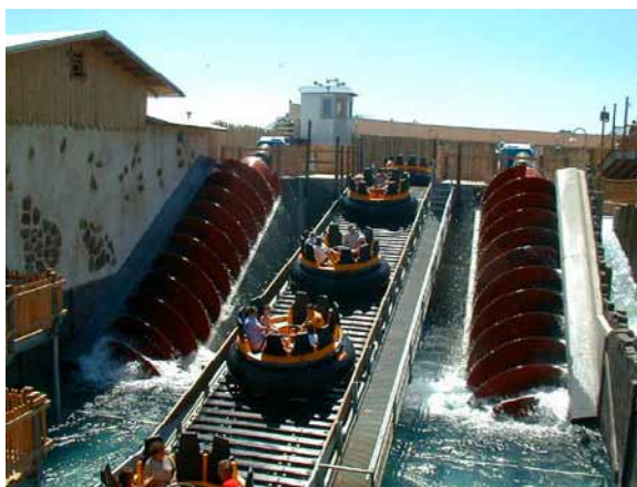
Fig. 5 Archimedian Screws installed in a theme park (29)
