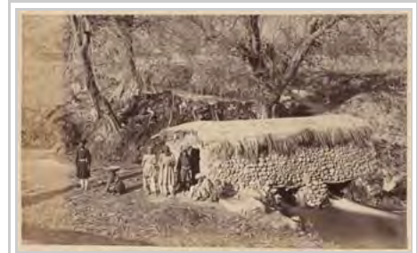
An Afghan water mill photographed during the Second Anglo-Afghan War (1878-1880). The rectangular water mill has a thatched roof and traditional design with a small horizontal mill-house built of stone or perhaps mud bricks
