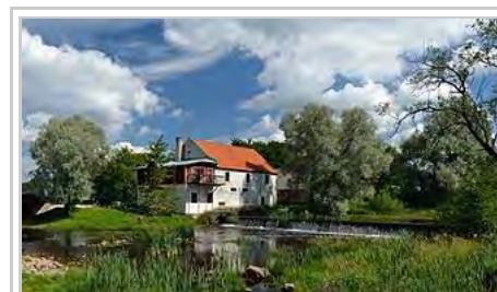
Former watermill in Kohila, Estonia
