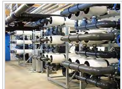
Ultrafiltration for a swimming pool
