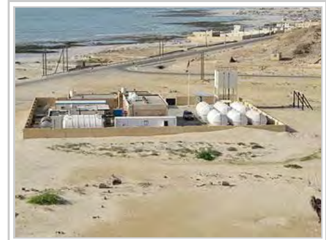
Modern Water's containerised forward osmosis desalination plant at Al Khaluf, Oman
