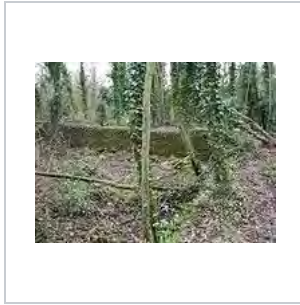
World War II aircraft revetments made of sandbags, as seen decades later in 2009.
