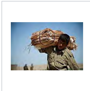
An Afghan Local Police officer carries a bundle of empty sandbags during a checkpoint construction project
