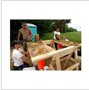
Improved method of sandbag filling.
