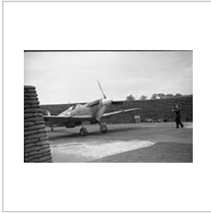
Sandbagged aircraft revetment
