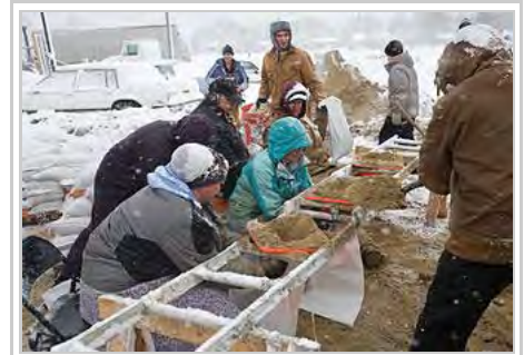
Sandbags being filled using a ladder on sawhorses with traffic cones as chutes or funnels, Moorhead, Minnesota, 2009.
