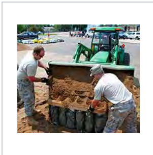
Filling multiple sandbags with a front-end loader.
