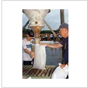
Manual filling of sandbags from a hopper or silo
