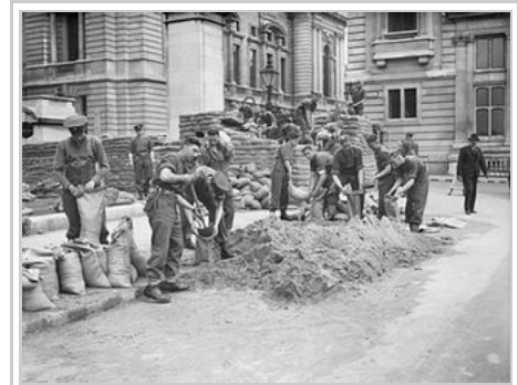
Troops from the Grenadier Guards constructing sandbag defences around government buildings in Birdcage Walk, London, May 1940.
