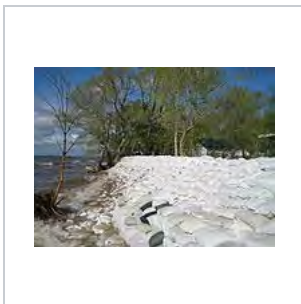
A sandbag wall to limit erosion, wave damage and flooding
