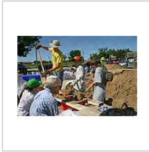
Sandbags being filled using improvised methods, lumber and traffic cones as chutes, Iowa City, Iowa, 2008.
