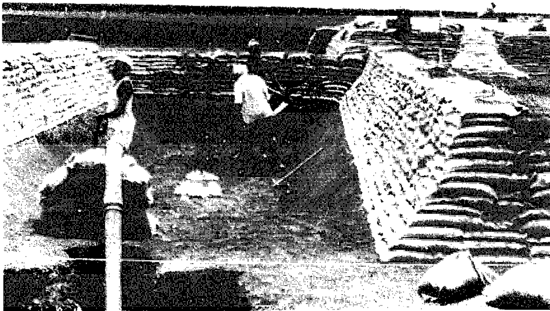
Figure 2.2: Horizontal flow-roughing filter under construction, Fau, Sudan (photo IRCWD)
