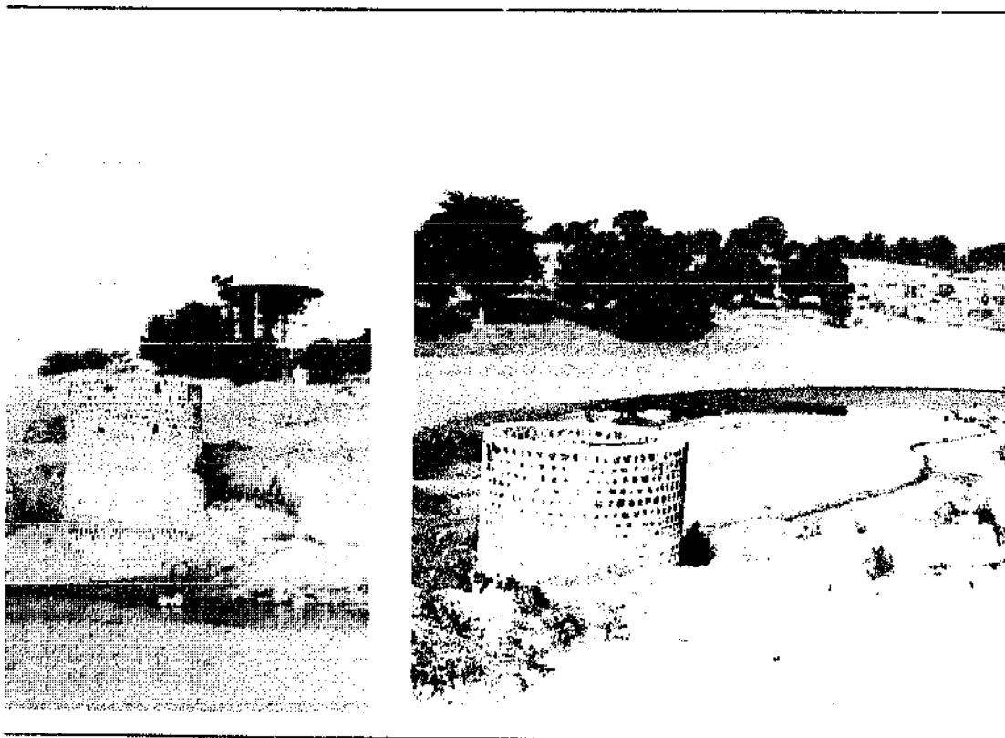
Figure 2.1: River bed filtration, collection well, Borujwada, India
