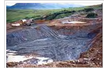
Settling pond under construction, Blue Ribbon Mine, Alaska
