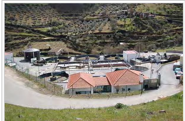
A sewage treatment plant in northern Portugal.
