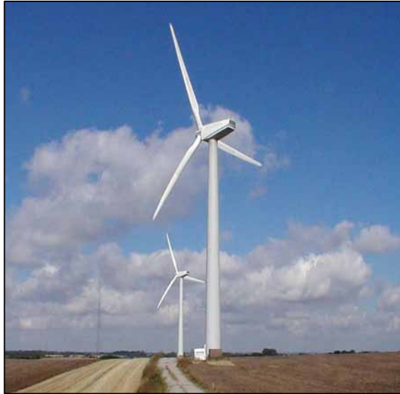
Figure B-1 The Norwin 46-ASR-600 kW turbines Ørsted 2 (in front) and Ørsted 1 used in the measuring program. The wagon containing the measuring equipment is seen besides Ørsted 2, and the measuring mast is seen to the left of the road.
