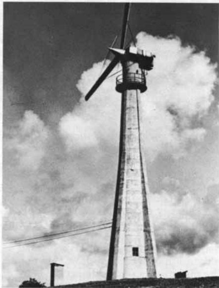
Figure 6. Research windmill of J. Juul, utility company SEAS, at the island Bogø. Early 50s, 45 kW AC.
