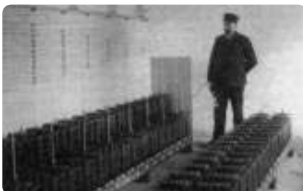
The battery store room of a wind power plant at the beginning of the 1900's • (H.C.Hansen: Poul la Cour)
