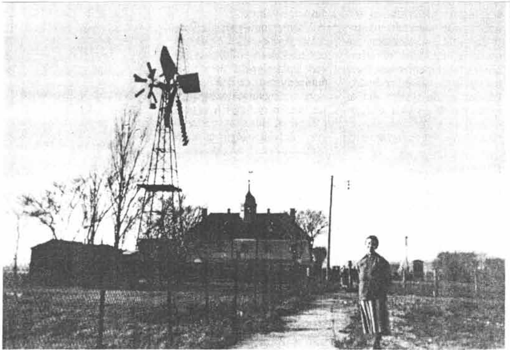
Wind-turbine of Type 1 - 1.5 built 1904. 10 kW DC Generator Tower height 17 m. Blade diameter 16 m. Sited in Copenhagen Harbour, in operation until 1957. This was a combined wind-turbine - petroleum spark ignition motor generator.
