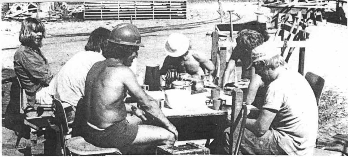
Tower-construction crew - Tvind Wind-Turbine - Summer 1975.
