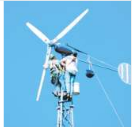
(Above) A remanufactured Jacobs is installed during an MREA workshop.
