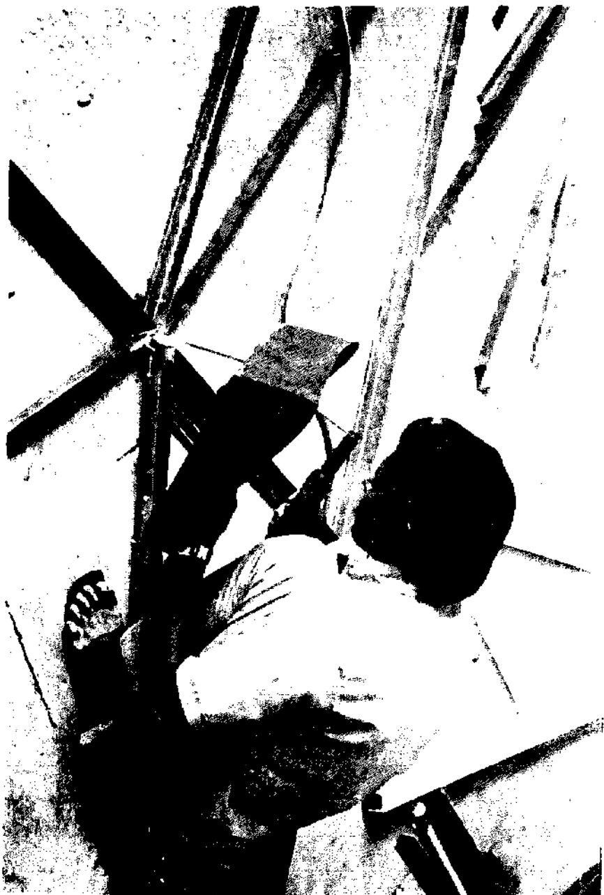
Part of tower half is composed and welded.
