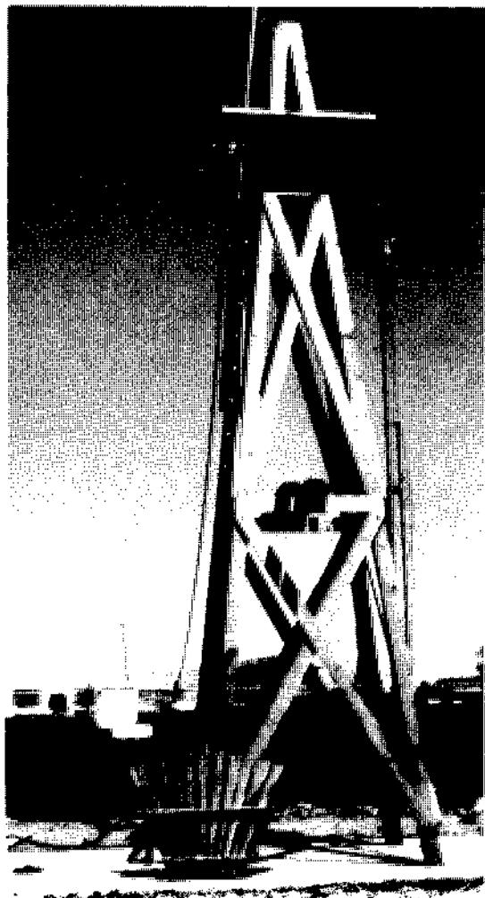
Figure 2.5 A 40-foot wooden windmill tower.
