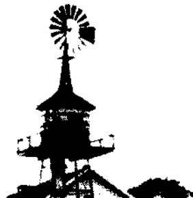
Figure 2.14. A windmill, storage, and pressure system, all on one tower.
