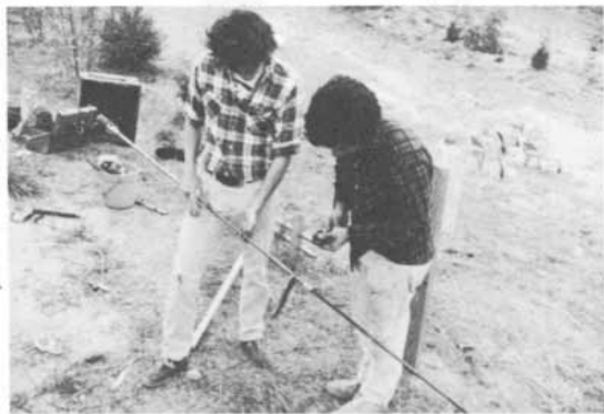
Figure 5.6. When attaching sections of pump rod, be sure to avoid bending the rod.
