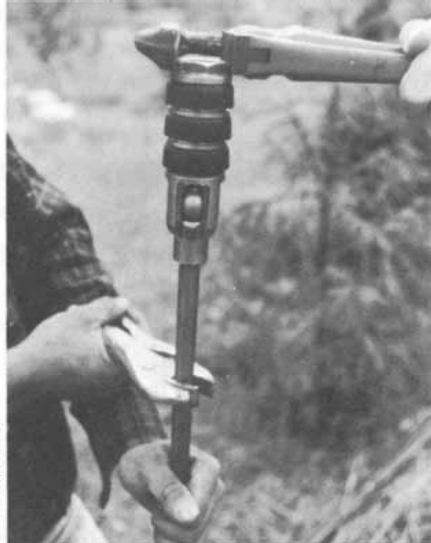
Figure 5.5. Attaching the plunger to the pump rod.
