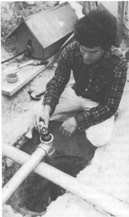
Figure 5.3. Seating the bottom check valve in an open top cylinder. Make certain that paper or cardboard protectors are removed from the ball valve.
