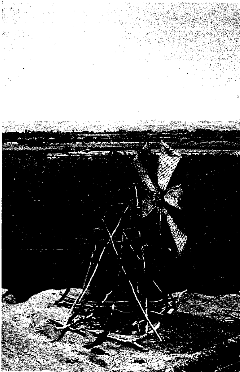
A wind pump made using village technology at Miramar, Peru.
