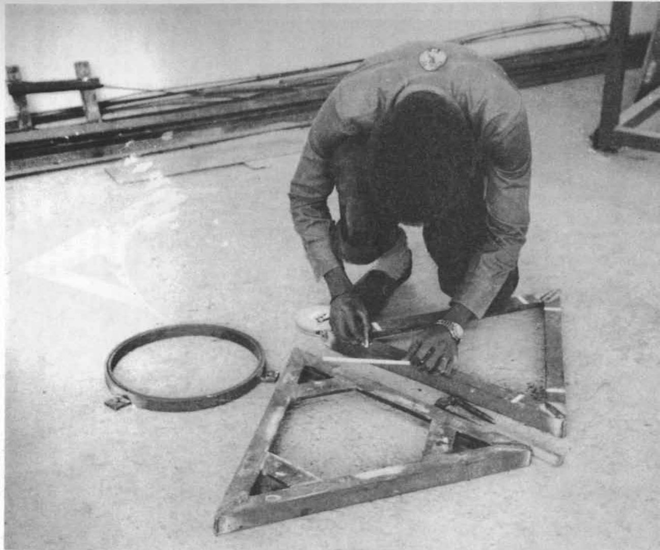
Making upper tower section frame.
