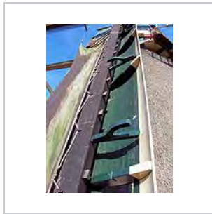
Close-up of Fok system with spread sailcloth
