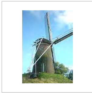
Ten Have sails open on one stock, common sails on the other, both with van Bussel system.
