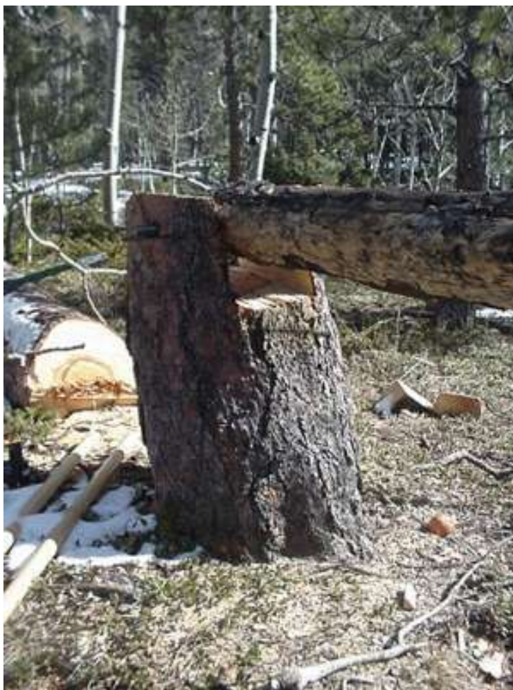
Hinged base made from tree stump
