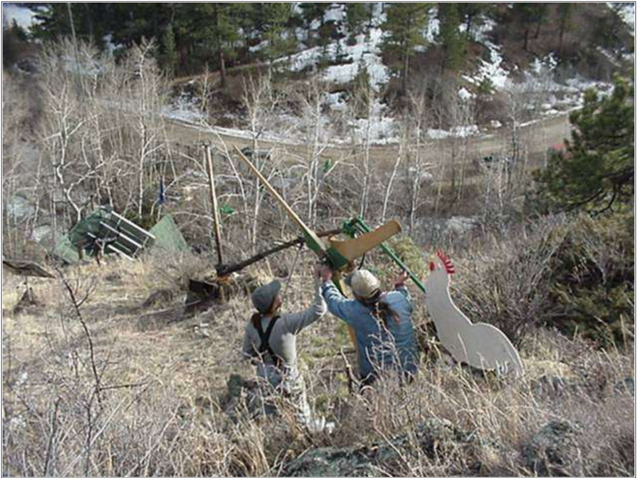
Here we are assembling the machine on the tower top.
