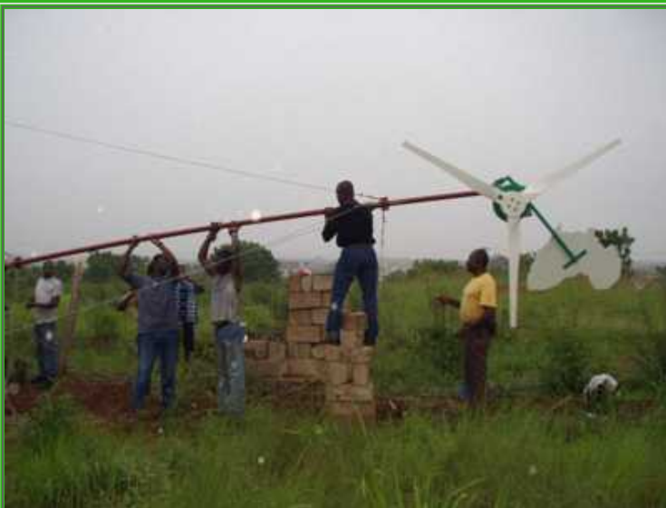
Wind turbine construction course in Ghana July 2004
