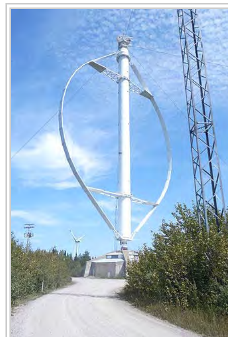
The world's tallest vertical-axis wind turbine, in Cap-Chat, Quebec
