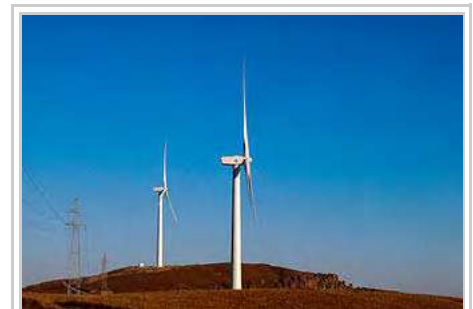
Onshore Horizontal Axis Wind Turbines in Zhangjiakou, China
