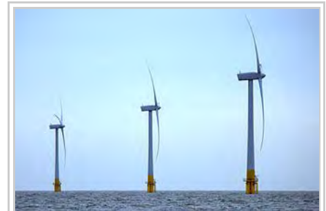
Offshore Horizontal Axis Wind Turbines (HAWTs) at Scroby Sands Wind Farm, UK
