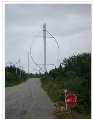
Éole, the largest vertical axis wind turbine, in Cap-Chat, Quebec, Canada
