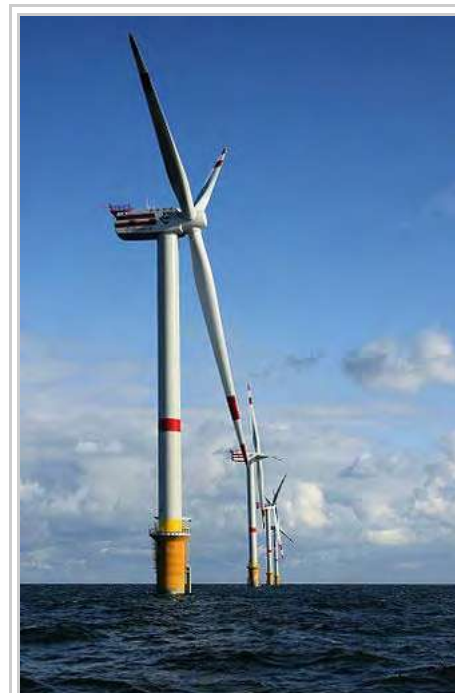
Offshore wind farm, using 5 MW turbines REpower 5M in the North Sea off the coast of Belgium.
