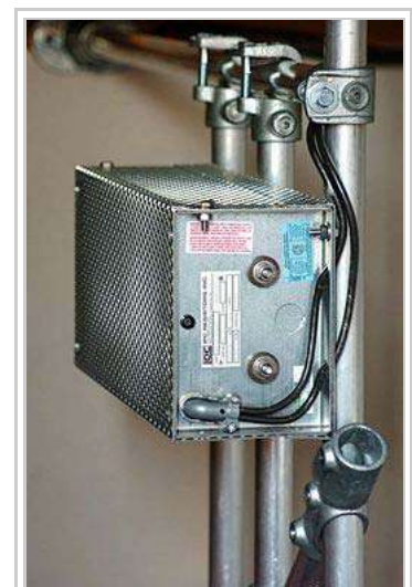
2kW Dynamic braking resistor for small wind turbine.
