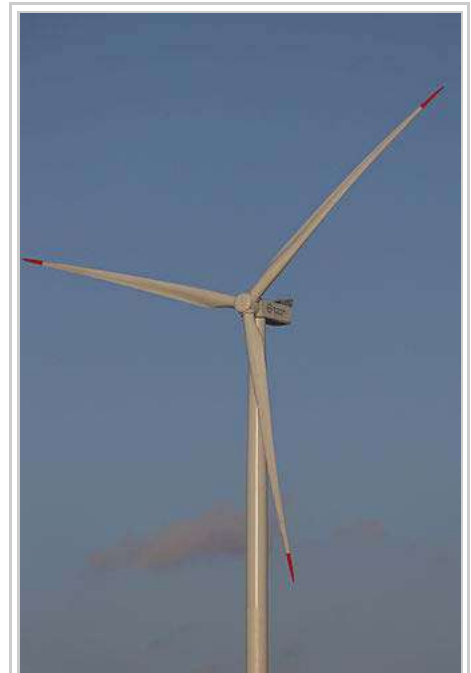
Several modern wind turbines use rotor blades with carbon-fibre girders to reduce weight.
