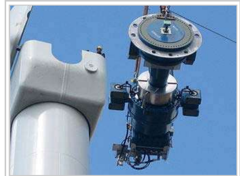
Gearbox, rotor shaft and brake assembly
