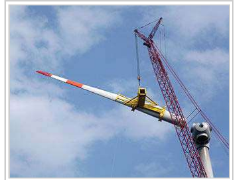
Liftra Blade Dragon installing a single blade on wind turbine hub. [83][84]
