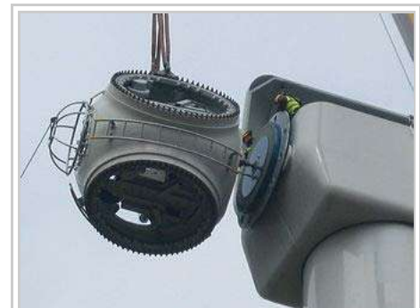
A Wind turbine hub being installed
