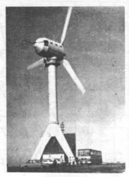
to operate connected to the grid (system) has two generators operating in oversynchronous state.
