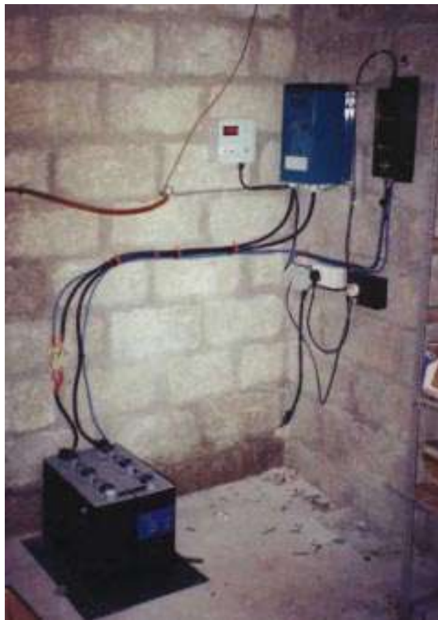
Photo 12: A traction battery from a forklift truck can be deeply cycled over 1000 times (Hugh Piggott, UK)
