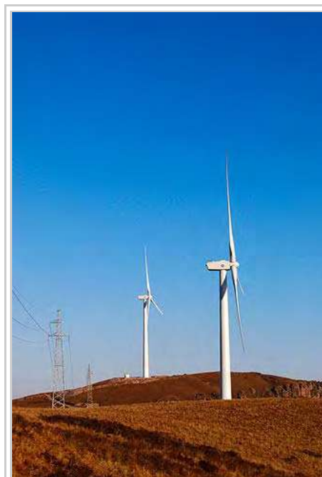
A group of wind turbines in Zhangjiakou, China
